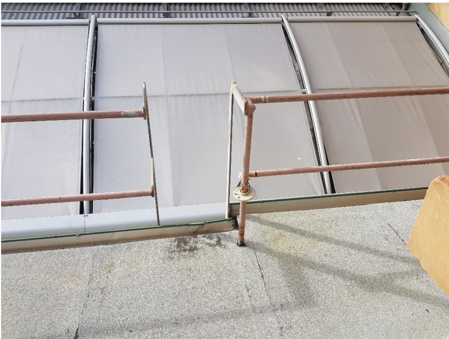
Figure 6: Balustrade North West
