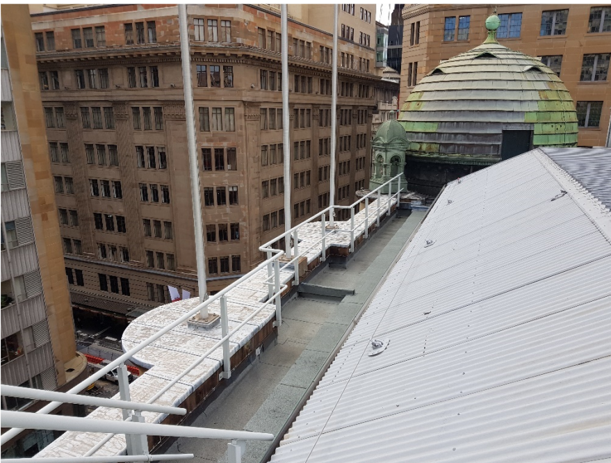
Figure 2: Flag Poles North End
